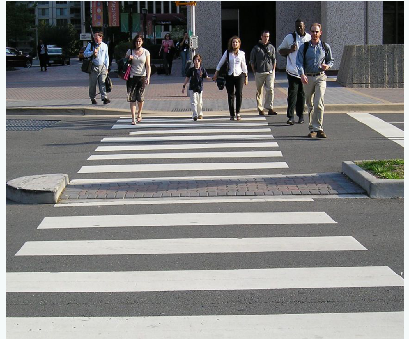
Continental crosswalks enhance pedestrian visibility by clearly demarcating the pedestrian crossing area. Additionally, pedestrian refuge islands break up raised center roadway medians to create a safe stopping point for pedestrians.
