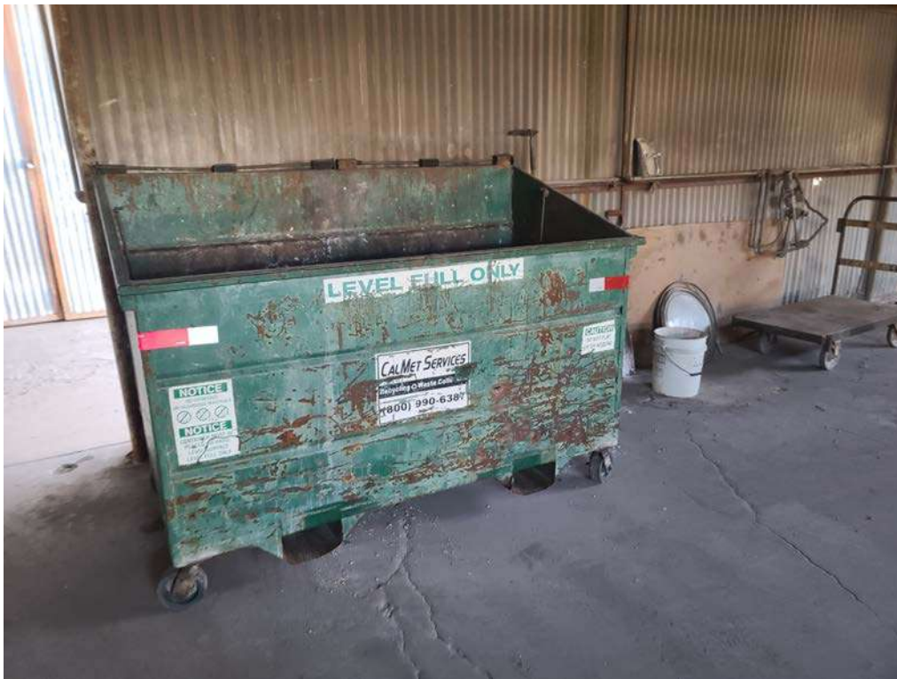
Photo 9: View of empty waste dumpster in building.
