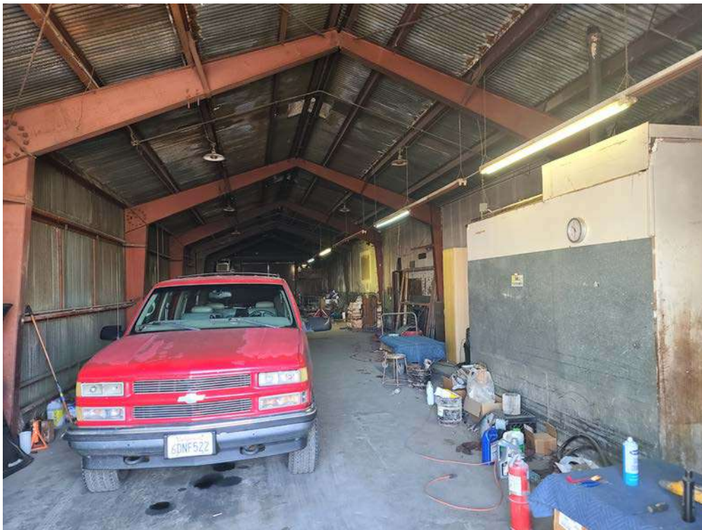
Photo 4: View of interior of building 3.
