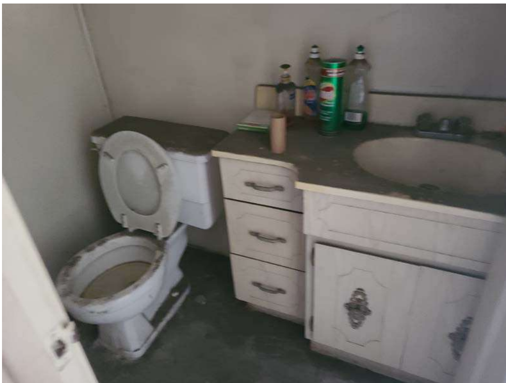
Photo 12: View of typical restroom in building.
