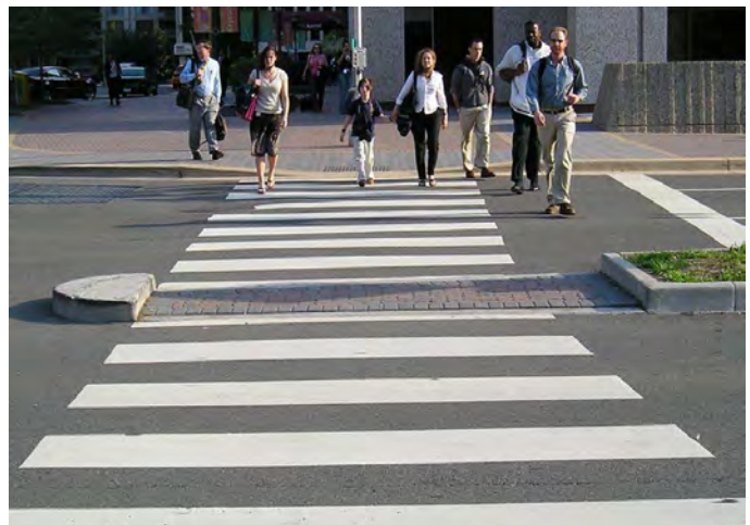
Continental crosswalks enhance pedestrian visibility by clearly demarcating the pedestrian crossing area. Additionally, pedestrian refuge islands break up raised center roadway medians to create a safe stopping point for pedestrians.
