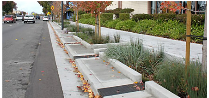
Flow-through planters along the street provide space for on-street parking to have space to enter/exit
