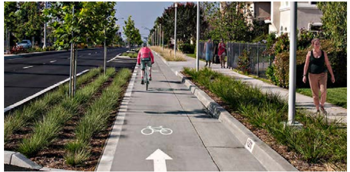
Bioswale protected bicycle lane with no curb facing the bicycle lane to allow stormwater infiltration
