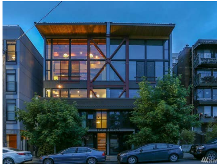
Stacked flats apartment building that creates walkable urban fabric along with adjacent buildings of similar scale
