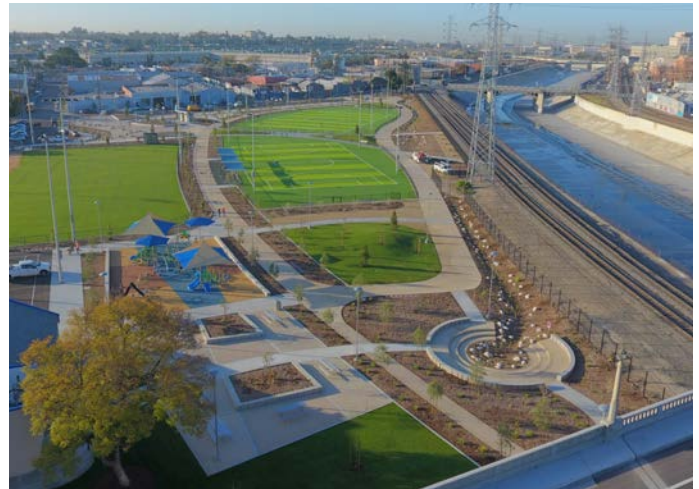
Albion Riverside Park, Lincoln Heights, Los Angeles provides an example of a different landscape areas acting as a cap park from an amphitheater to soccer field.
