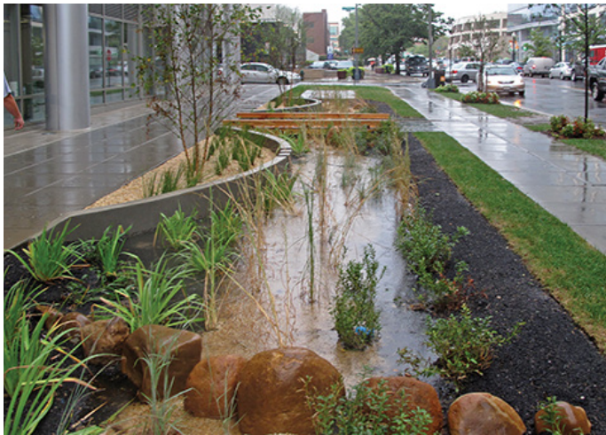
A rain garden during a rainstorm that is wider than a typical sidewalk parkway
