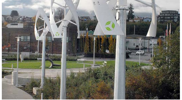
Example of small wind turbines that can act as wayfinding elements, public art, or placed on buildings
