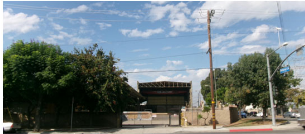
Facing east along Petterson Lane
