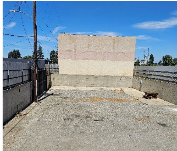
Interior of project site, facing north.
