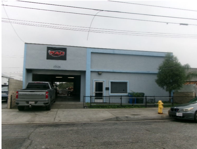
The west side of the property, adjacent to Vermont Ave
