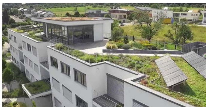
Building with a green roof as resident amenity space and solar panels
