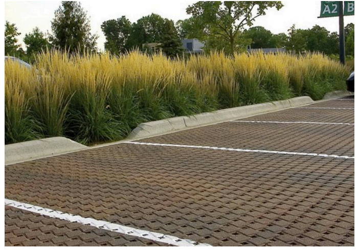
Integrating bioswales with permeable pavement areas, this example for a surface parking lot
