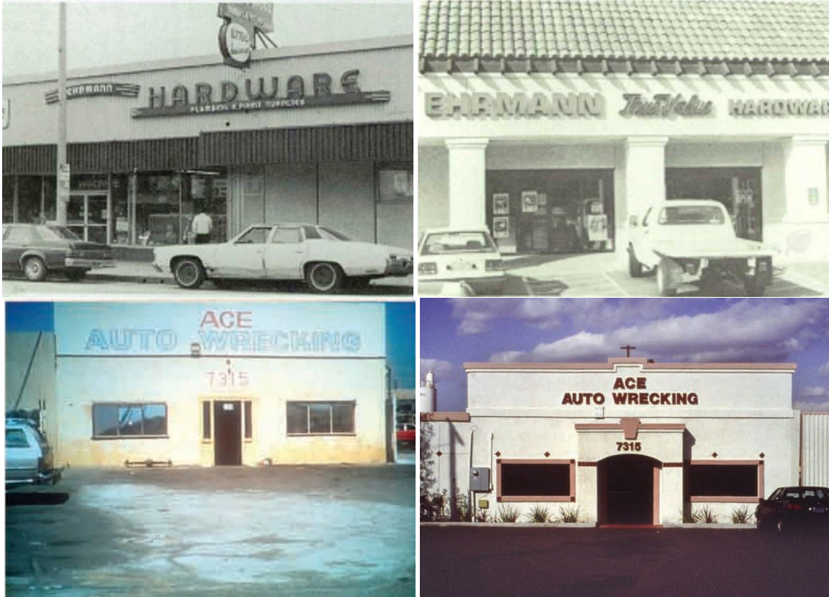
Before and after renovation/relocation projects for Ehrmann's Hardware (top) and Ace Auto Wrecking (bottom). City of Paramount.
