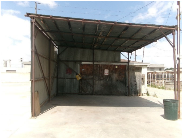
Existing building, to be demolished.
