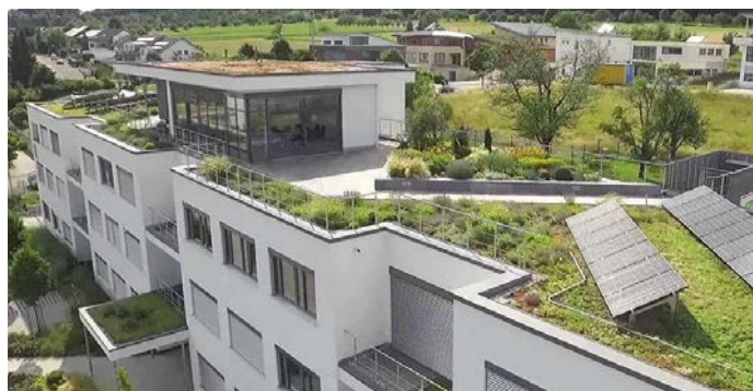
Building with a green roof as resident amenity space and solar panels
