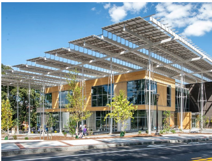
Flex building with solar panels that extend outside the footprint of the building, creating a publicly accessible shaded entry plaza
