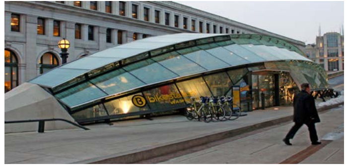
Stand-alone bicycle parking hub and repair station
