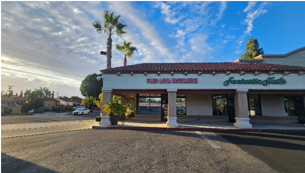
Front view of the tenant space.
