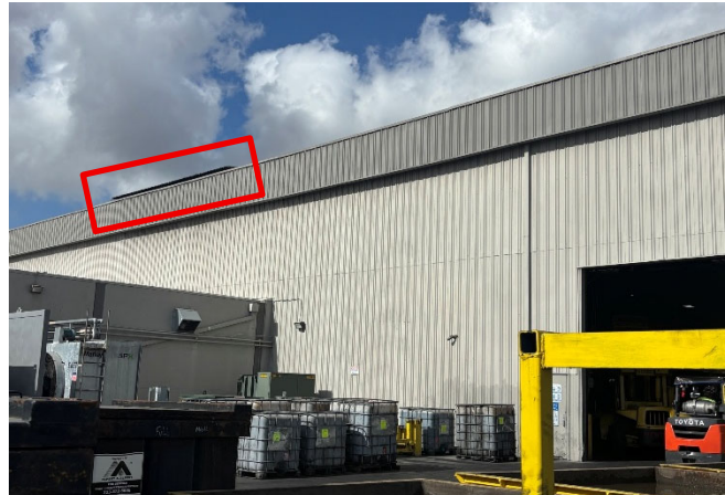
East side of building (showing existing roof opening)
