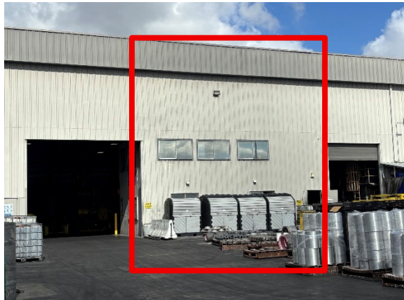
East side of building (proposed expansion area)
