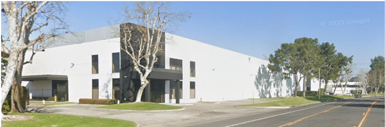
View looking northwest at the subject building from Orange Avenue (Feb. 2025, Google Street View).
