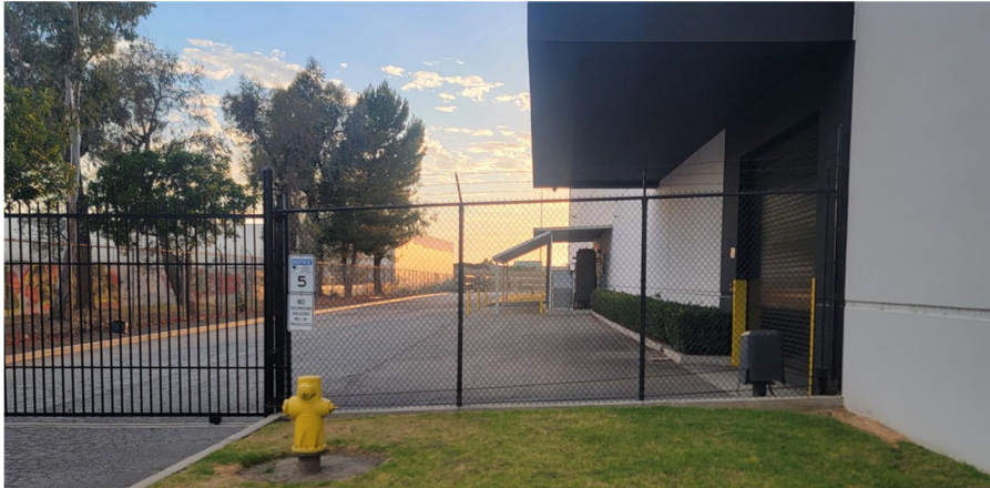
View of chain link fencing with barbed wire on south side of building
