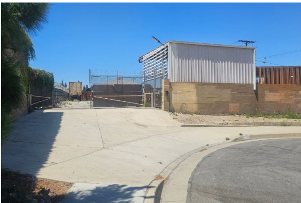
Front/north view of the subject site.
