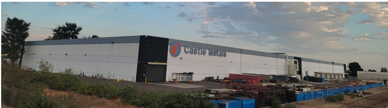
View looking southeast from Los Angeles River Path
