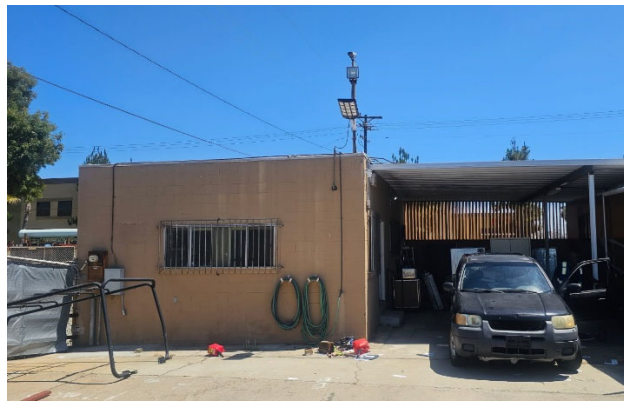
South-facing view of the existing storage building.
