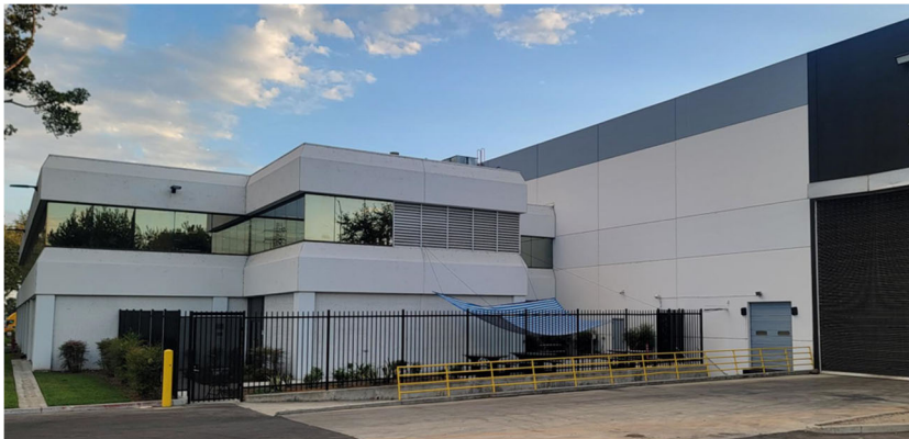
View looking south at office area at north side of the building
