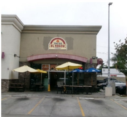
Front of the existing restaurant Facing Rosecrans Avenue
