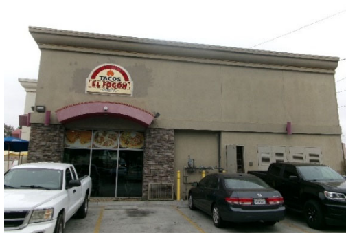
Side view of existing restaurant facing Garfield Avenue
