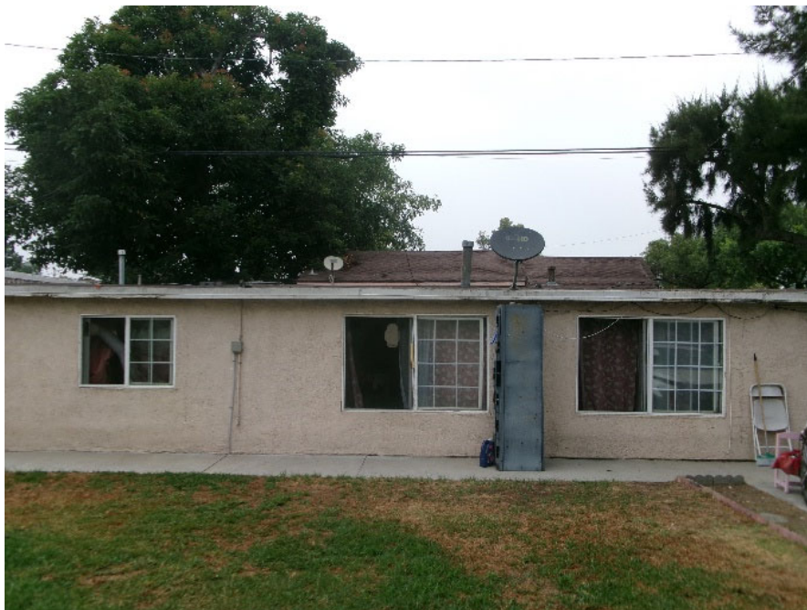
Project site from south point of view.
